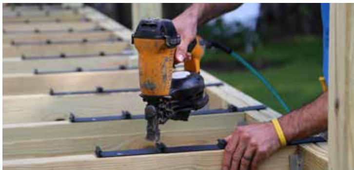
Position the end of each clip strip at chalk line and nail strips to each joist with side tabs tight against the same side of the joist.
