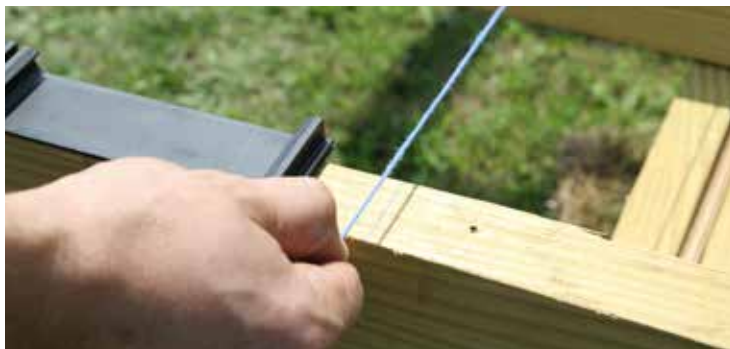
Snap a chalk line across the deck joists at a mark measured 21 5/8" (549 mm) (for 1" board overhang) from the outer edge or rim joist.
