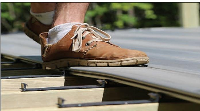
Position boards along each row of clips and step down or use a mallet on the board at each joist location to secure it into place.
