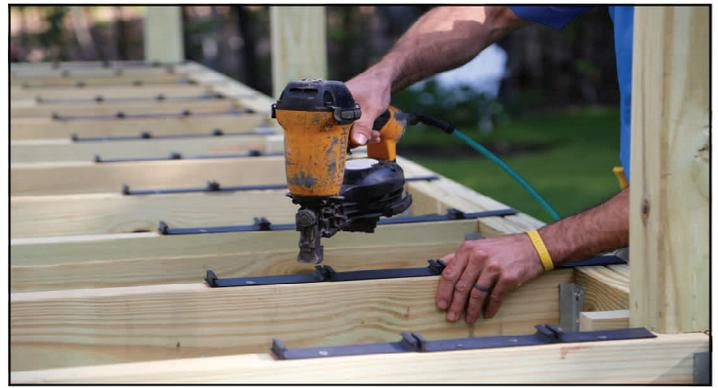
Position the end of each clip strip at chalk line and nail strips to each joist with side tabs tight against the same side of the joist .
