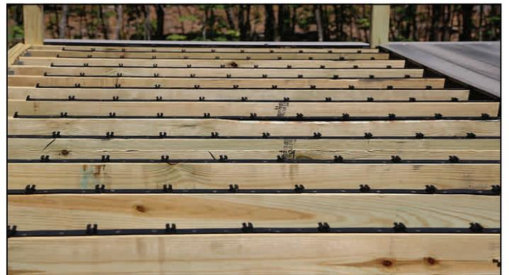
Strips may be installed on joists all at once prior to installing decking or one row at a time for elevated decks.
