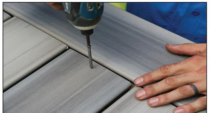
Align and secure interior boards with composite deck screws located at one end of each board (min. of 5/8" (16 mm) from board edge)
