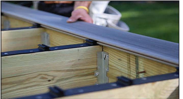
Slide starter board tightly into first set of clips and secure with composite deck screws along the outer edge of board.
