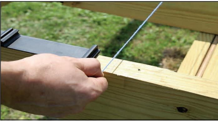
Snap a chalk line across the deck joists at a mark measured 22" (559 mm) (for 1" board overhang) from the outer edge or rim joist
